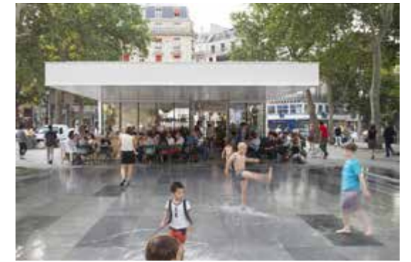
A pavilion building which creates interest and activity, busy through the day and into the evening
